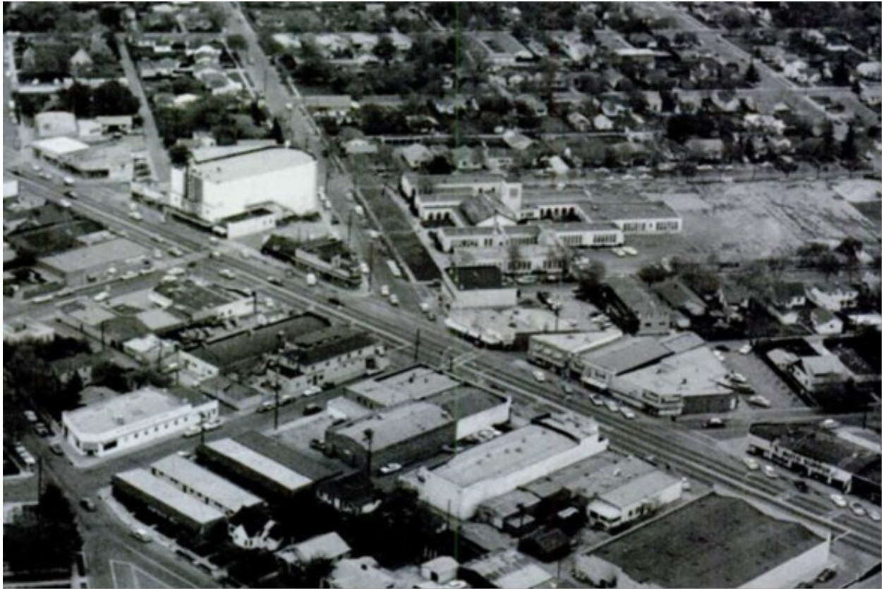
Figure 12 Aerial view from the west, 1950s. Ehrenreich-Risner, 30.
